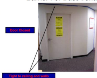
Barrier For Dust Control
