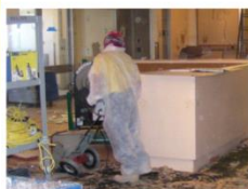
Use Of Coveralls During Demolition
